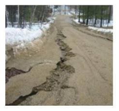
Severe erosion like this could have been prevented with a properly sized ditch.
